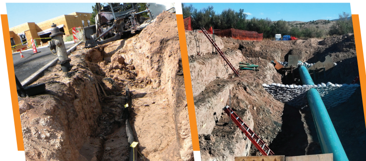
Kinder Morgan carbon dioxide pipeline construction project near Artesia.
